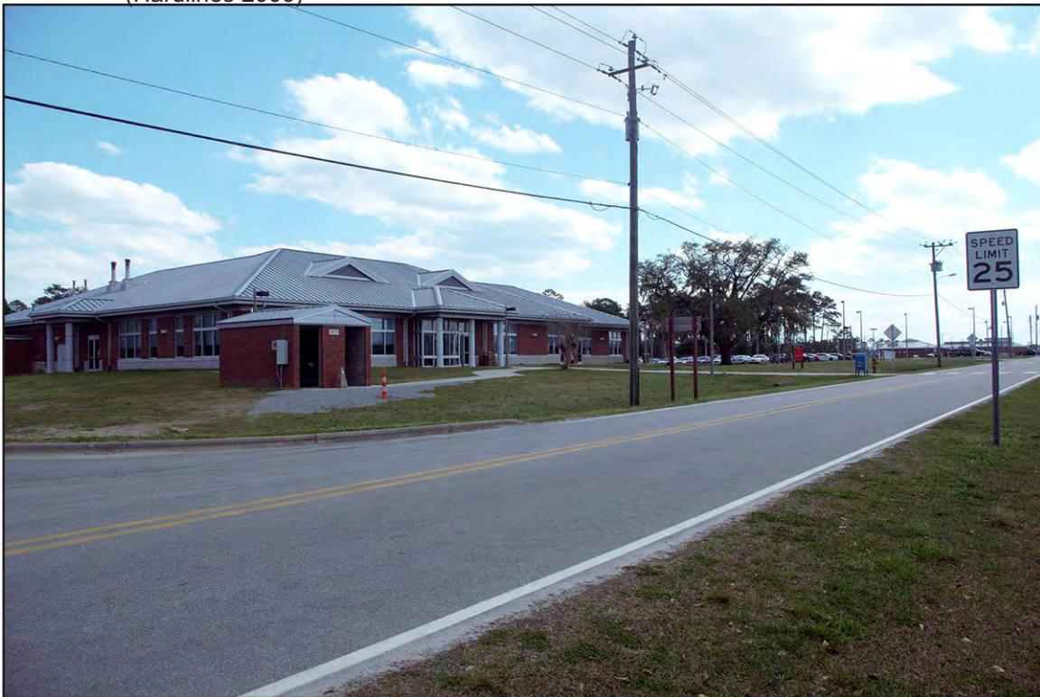
PLATE 25: Range Road, Looking Southeast Toward Recently Constructed MARSOC Dining Facility in the Location of the Former Family Officers' Quarters, Stone Bay Rifle Range Historic District, Camp Lejeune, North Carolina
