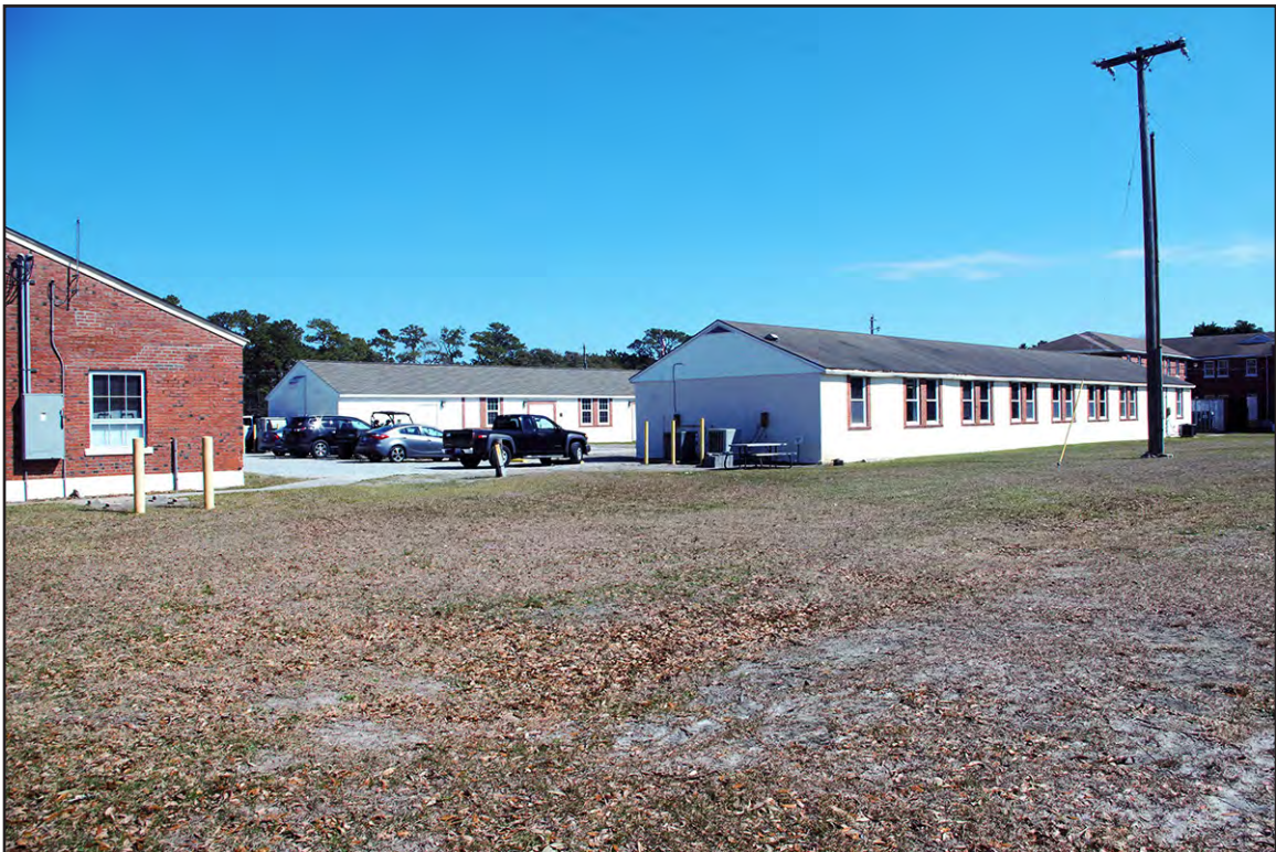
PLATE 10: Looking Northeast Toward RR50 and RR51 Classroom Buildings, Stone Bay Rifle Range Historic District, Camp Lejeune, North Carolina
