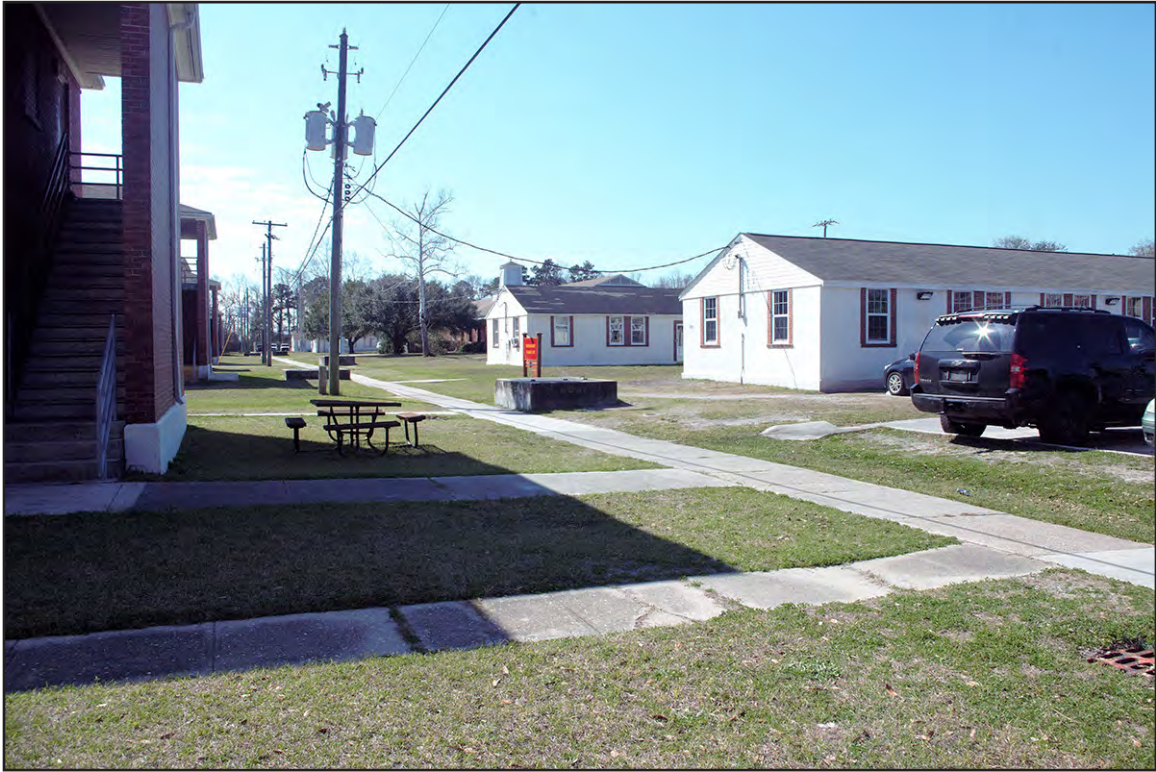
PLATE 11: Looking South Toward Barracks Buildings and RR51, Stone Bay Rifle Range Historic District, Camp Lejeune, North Carolina (Hardlines 2006)
