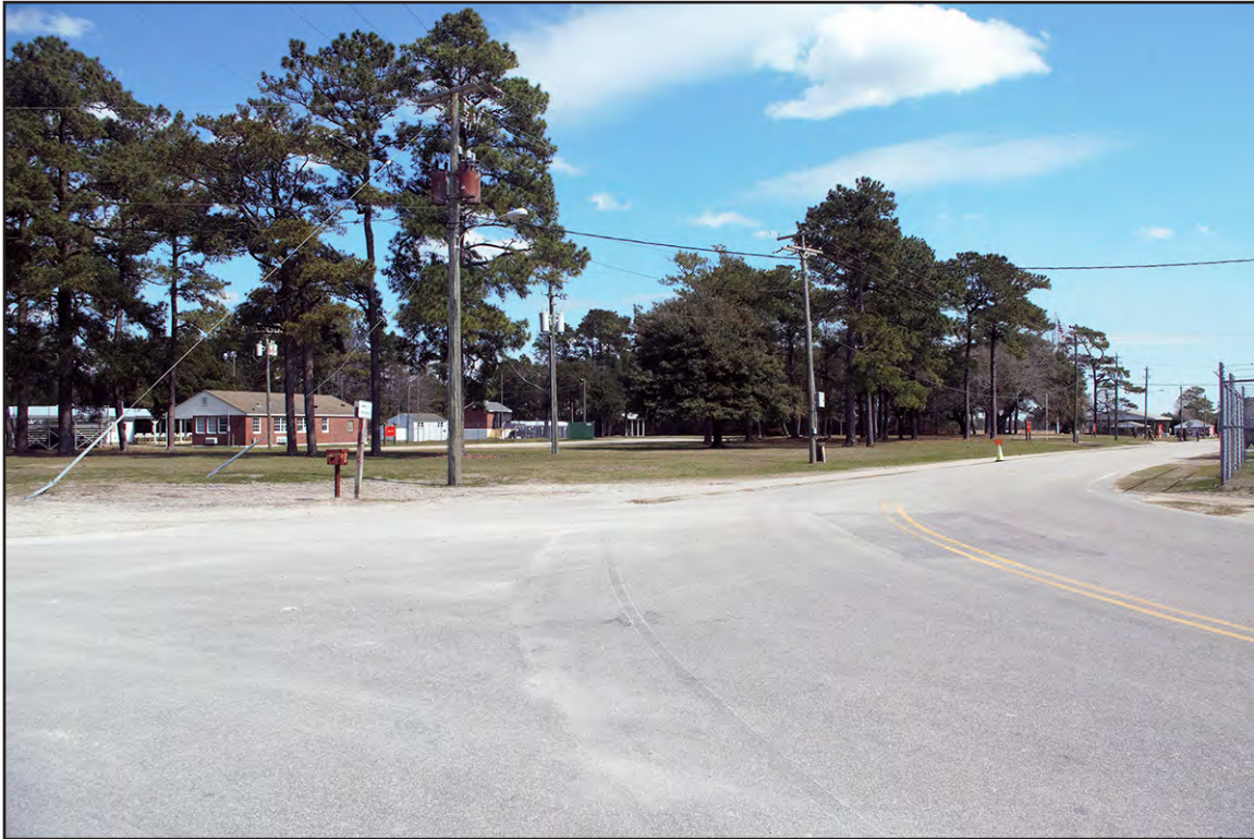
PLATE 1: Range Road, Looking Northeast Toward Pistol Range, Stone Bay Rifle Range Historic District, Camp Lejeune, North Carolina
