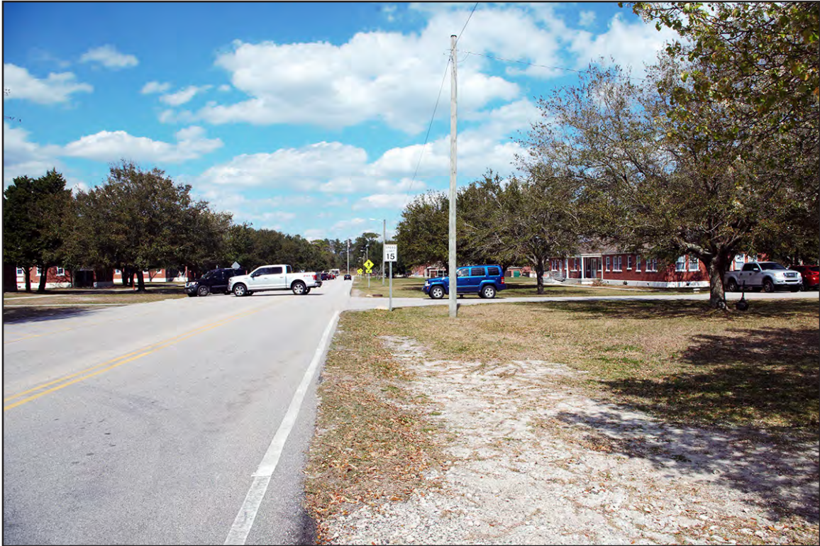
PLATE 13: Facing North on Range Road with Administrative and Support Buildings on Right and Barracks on Left, Stone Bay Rifle Range Historic District, Camp Lejeune, North Carolina
