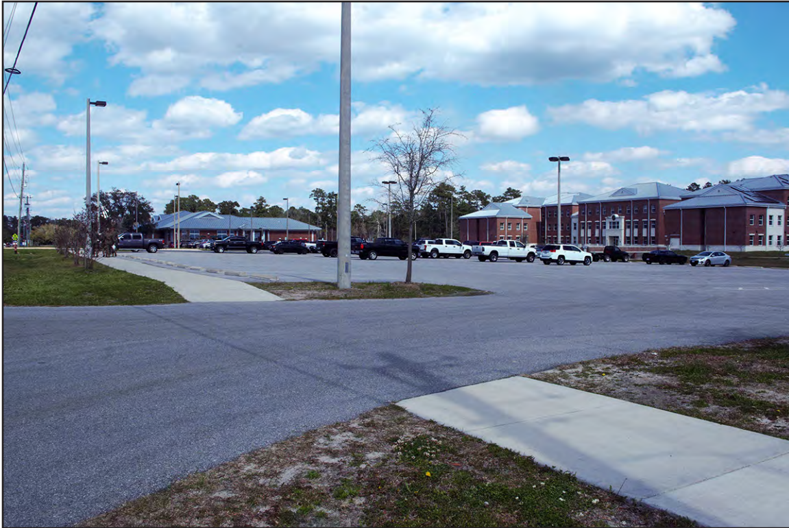
PLATE 26: Newly Constructed MARSOC BEQ and Dining Facilities, Looking Northeast, Stone Bay Rifle Range Historic District, Camp Lejeune, North Carolina
