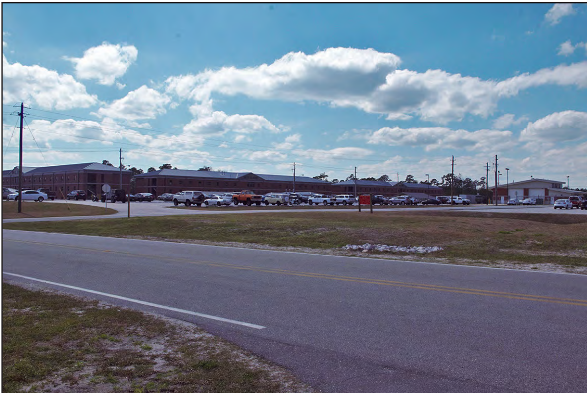
PLATE 7: Looking Southwest Across Range Road at the Southern End of the Stone Bay Rifle Range Historic District, Camp Lejeune, North Carolina
