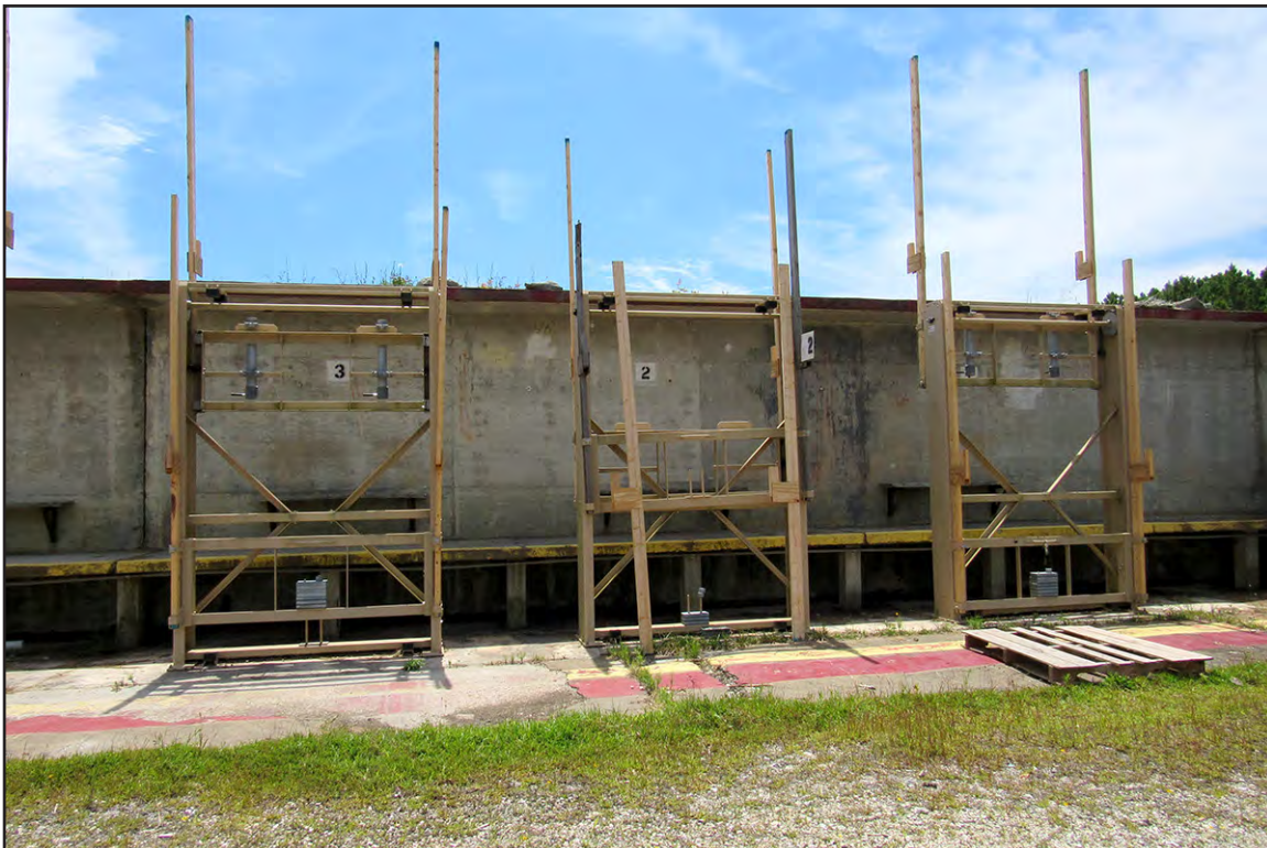
PLATE 21: Range Bravo, Detail of Concrete Wall and Pit with Butts, Looking South, Stone Bay Rifle Range Historic District, Camp Lejeune, North Carolina
