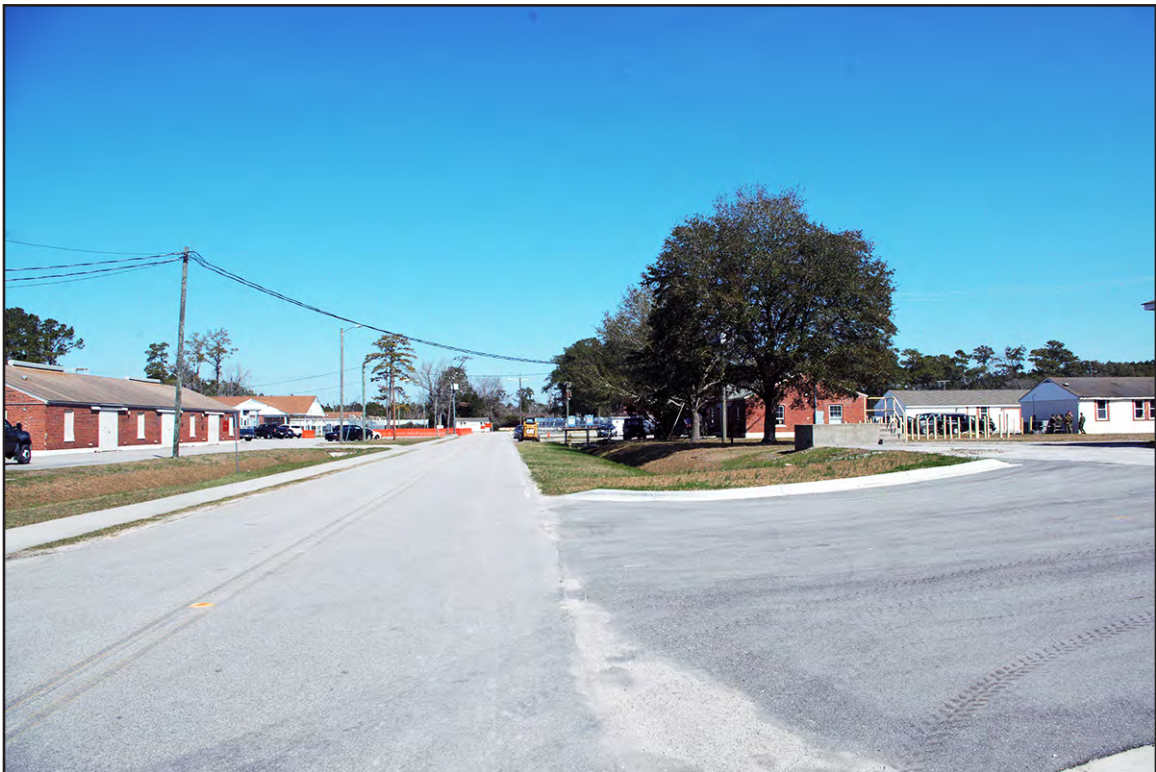
PLATE 14: Support Buildings and Battalion Warehouses Along Powder Lane, Facing North, Stone Bay Rifle Range Historic District, Camp Lejeune, North Carolina
