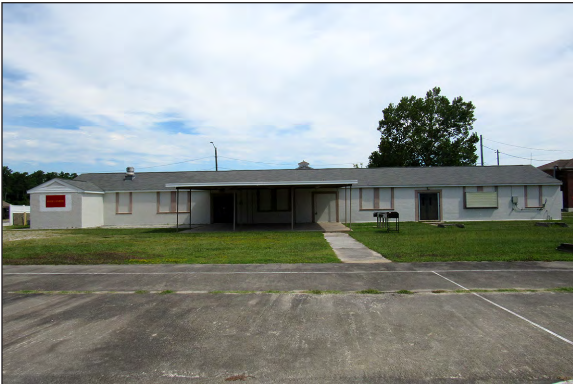
PLATE 30: RR49, Looking North, Stone Bay Rifle Range Historic District, Camp Lejeune, North Carolina
