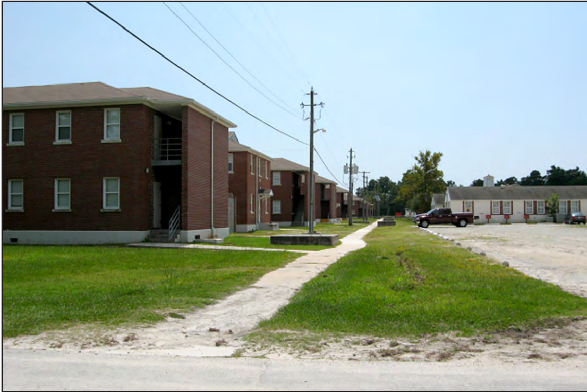
PLATE 29: Looking South Toward Barracks Buildings and RR51, Stone Bay Rifle Range Historic District, Camp Lejeune, North Carolina (Hardlines 2006)
